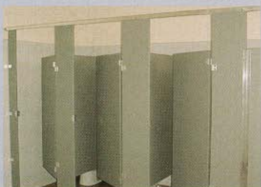
Mecklenburg County, Va. school district washroom improvements.
