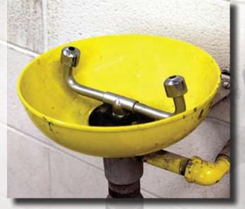
plumbed with tepid water, they may be hesitant to use an emergency shower or eyewash. Therefore, when an injured person uses a combination unit in an extreme environment, water temperature should be of the utmost concern.
