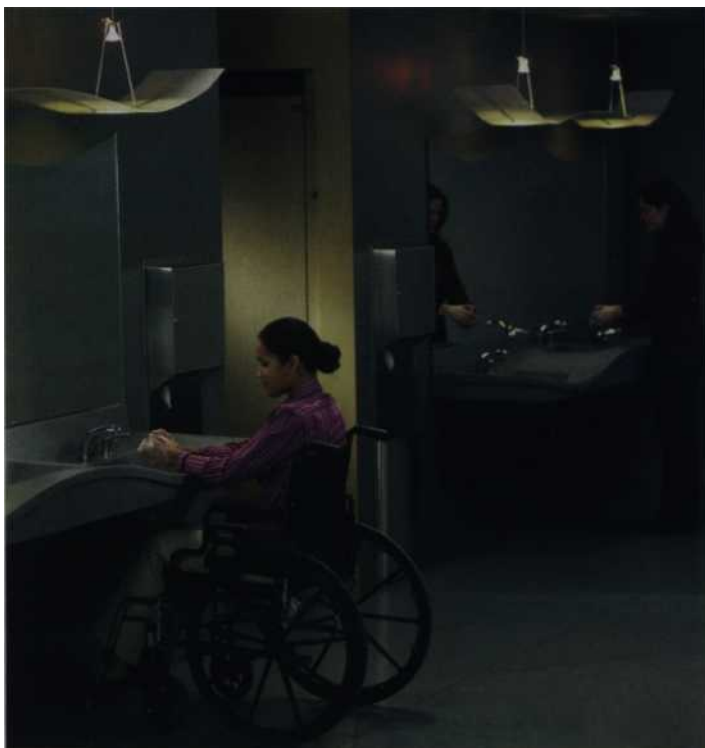
This is a multi-height lavatory system in use.
