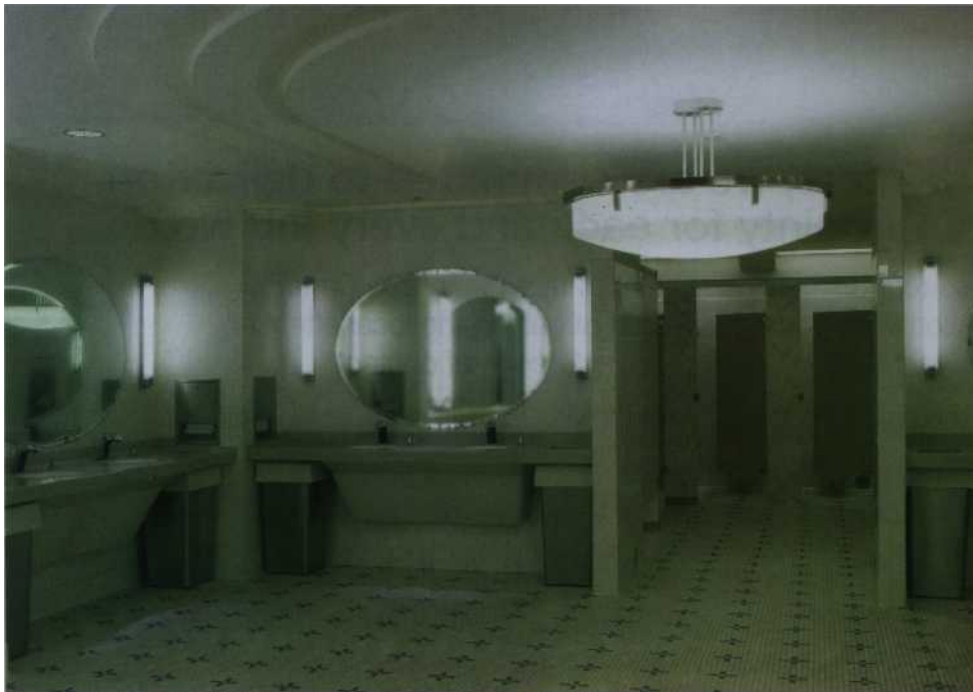
This is an ADA-compliant washroom at a Walt Disney World venue where trash cans were integrated into the lavatory units.
